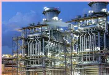
A top-tier gas-fired power plant in Singapore
