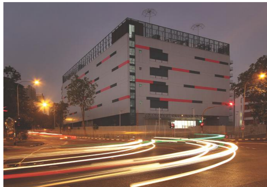
DataCentre One completed construction of 1-Net North and handed over the premises to the client.
