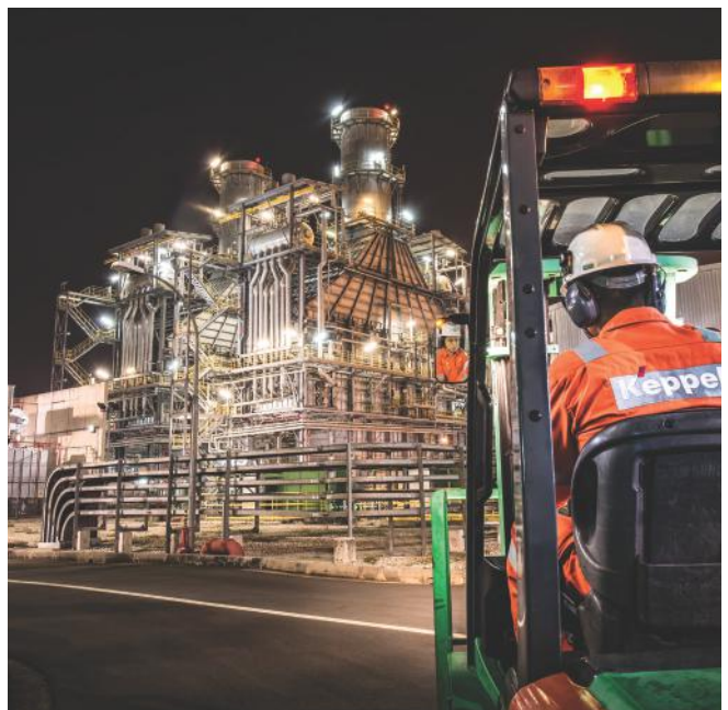
The KMC Plant has been operating since 2007 with a good track record of efficiency and reliability.
