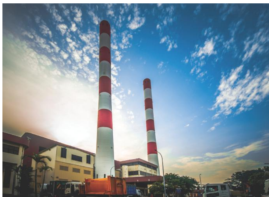
KIFM completed the capacity upgrade of the Senoko WTE Plant in September 2016.
