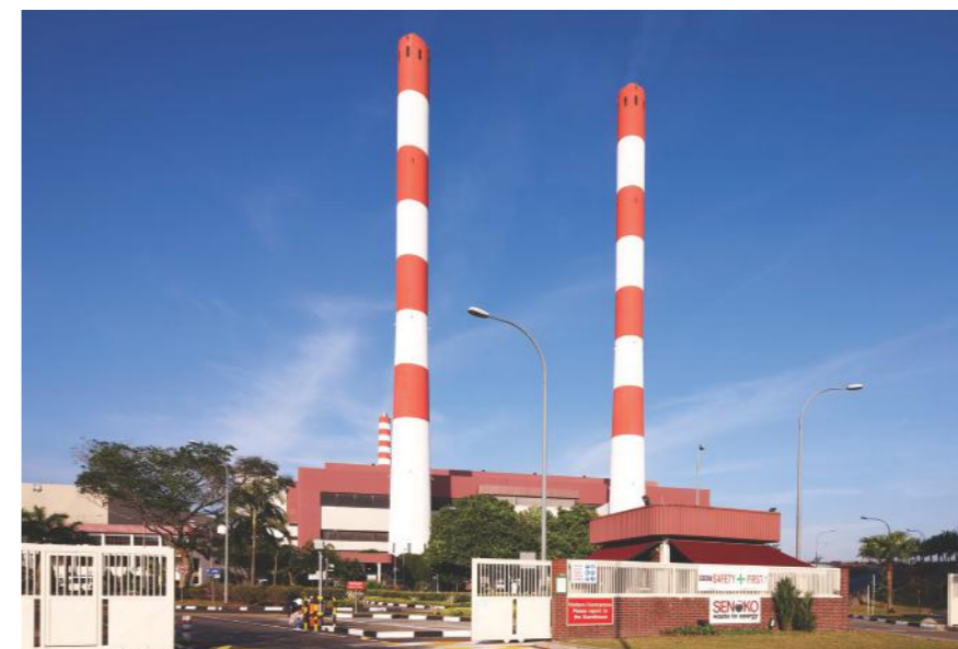
With the Senoko WTE Plant's contracted incineration capacity raised by 10% to 2,310 tonnes per day, the capacity payment from NEA has been correspondingly increased.
