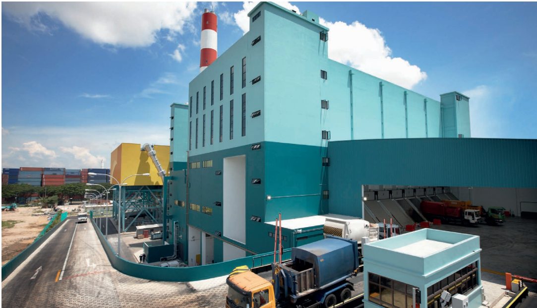
01 Keppel Seghers Tuas WTE Plant is equipped with two incinerator-boiler units capable of treating 800 tonnes of solid waste daily and one condensing turbine-generator offering a power generation capacity of 22 MW.
