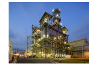
Keppel Merlimau Cogen Plant (KMC)
