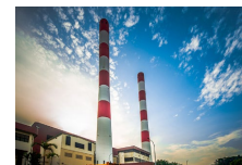
Senoko Waste-to-Energy (WTE) Plant
