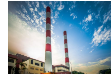
Senoko Waste-to-Energy (WTE) Plant
