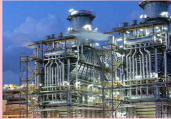
A top-tier gas-fired power plant in Singapore
