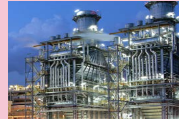
A top-tier 1,300MW gas-fired power plant in Singapore
